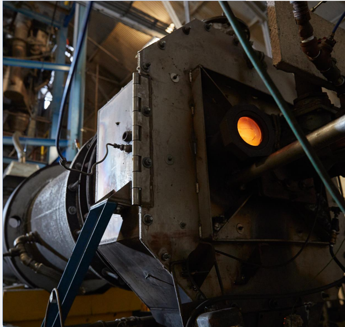
Calcining nodules at FLSmidth's facilities in Whitehall, Pennsylvania.
